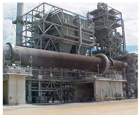
View of the 58 m long rotary kiln at Worsley.
