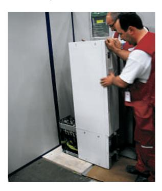
drive is wheeled over the pedestal and then locked into position 3.
