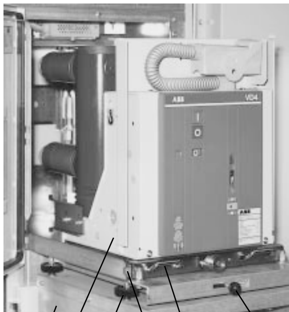
Figure 6/10: Withdrawable circuit-breaker part standing on service truck and secured in the catches
