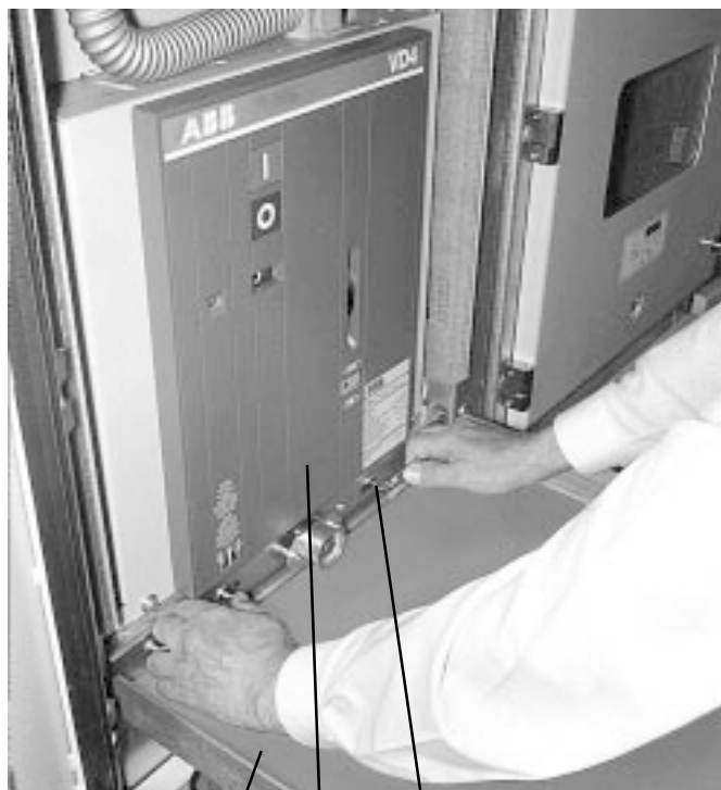
Figure 6/9: Service truck engaged with the panel. Withdrawable circuit-breaker part released for removal by moving the sliding handles inwards
