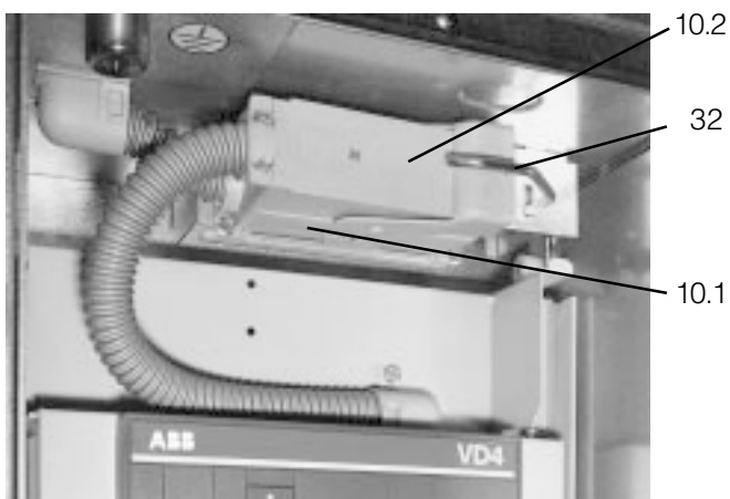
Figure 6/7: Control wiring plug connector blocked to prevent disconnection with the withdrawable breaker part in the service position
