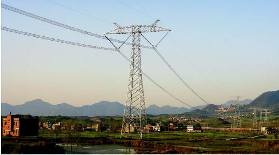
Figure 1. DC lines of Xiangjiaba-Shanghai UHVDC 800 kV project of SGCC in China
