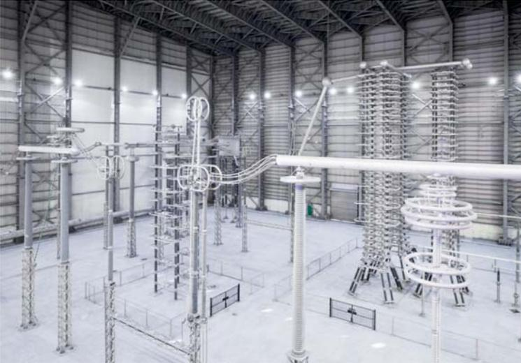
Figure 8. Indoor DC yard of an 800 kV UHVDC project.
