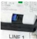
Displays the cause of the trip of the DS200 residual current breaker. Blue (residual current trip) or black (over-current trip indications).
