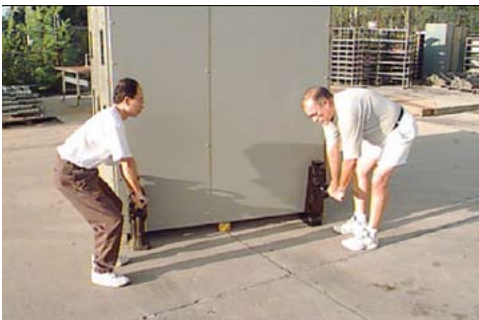
Figure 2. Position jacks under the front and rear corners, inside the shipping base.
