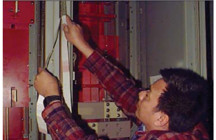
Figure 16. Install gasket material between shipping splits before bolting together.
