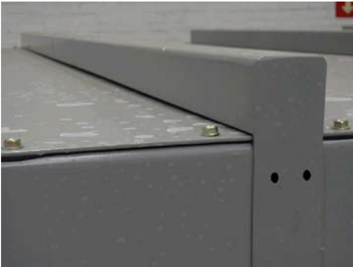
Figure 19. Loosely install the shipping split angle as shown.
