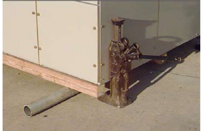
Figure 3. Raise the unit enough to position a roller under the shipping base.
