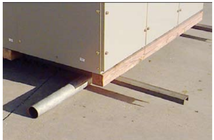
Figure 4. Position rails on rollers as shown for lateral moving.
