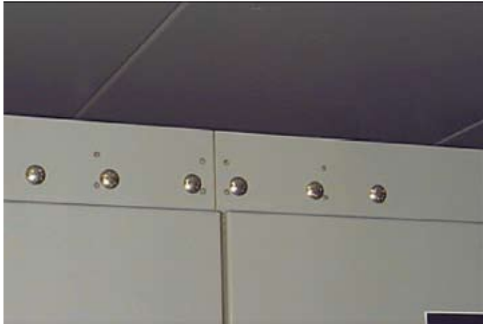
Figure 10. Secure plates and rails for a smooth and continuous transition between sections.
