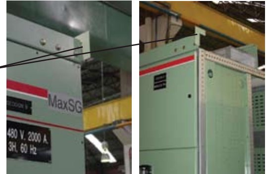
Figure 8. Remove the Carriage Stop and End Panel.
