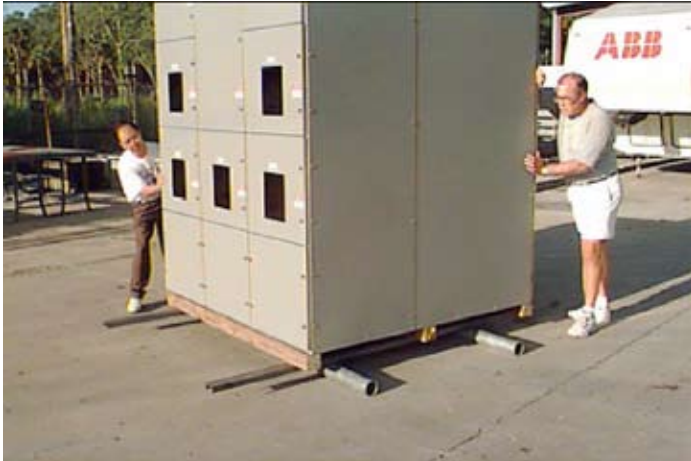
Figure 5. Carefully push the unit onto a third roller.
