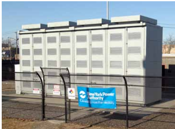
Battery storage facility at Long Island Bus depot.
