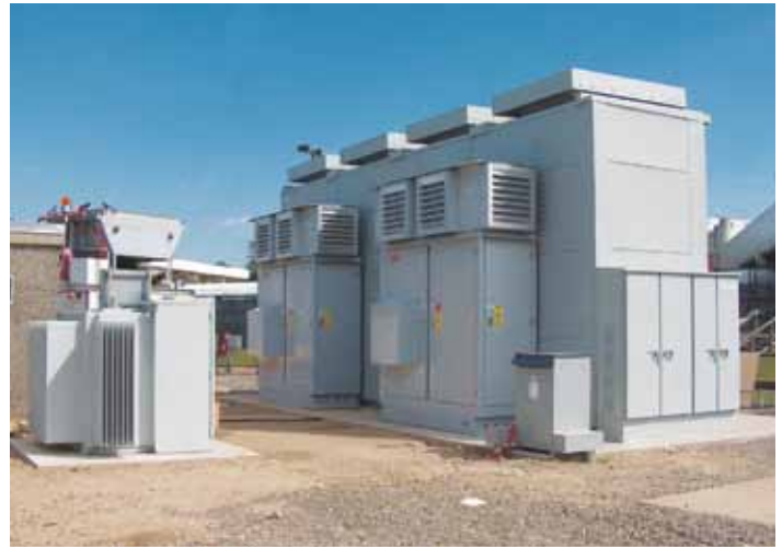
ABB's Power Conversion System (PCS), which converts energy for charging and discharging the battery system.
