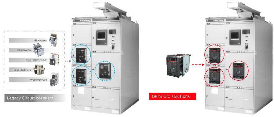
Switchgear with legacy circuit breakers
