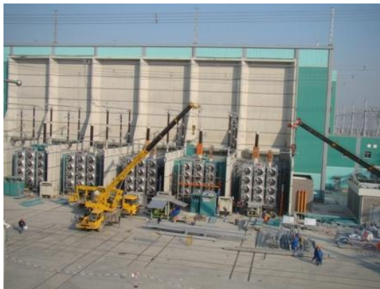
Figure 5. Converter transformers
