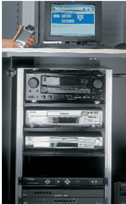
9 All technical functions (lighting, blinds, climate, audio and video) in the meeting room are controlled over the web.
