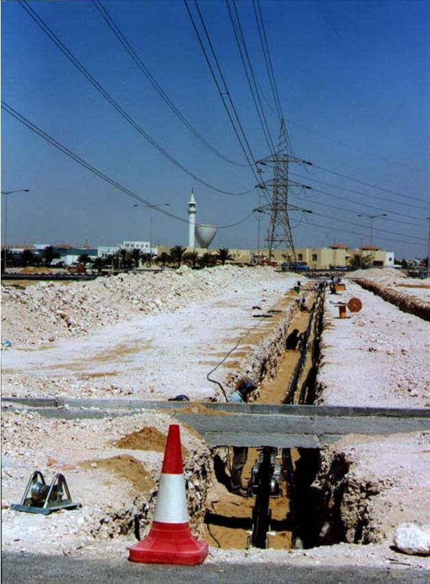
Figure 5: Example of cable laying in a corridor already used by OH-lines. AC PEX-cable in Qatar.
