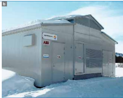
5 A MALTE prefabricated substation: old substation a , new substation b and interior of the new substation with a power transformer in the middle, high-voltage to the right, and medium-voltage and secondary equipment on the left c
