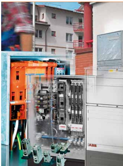
1 Devices close to the plug to provide safe electrical power
