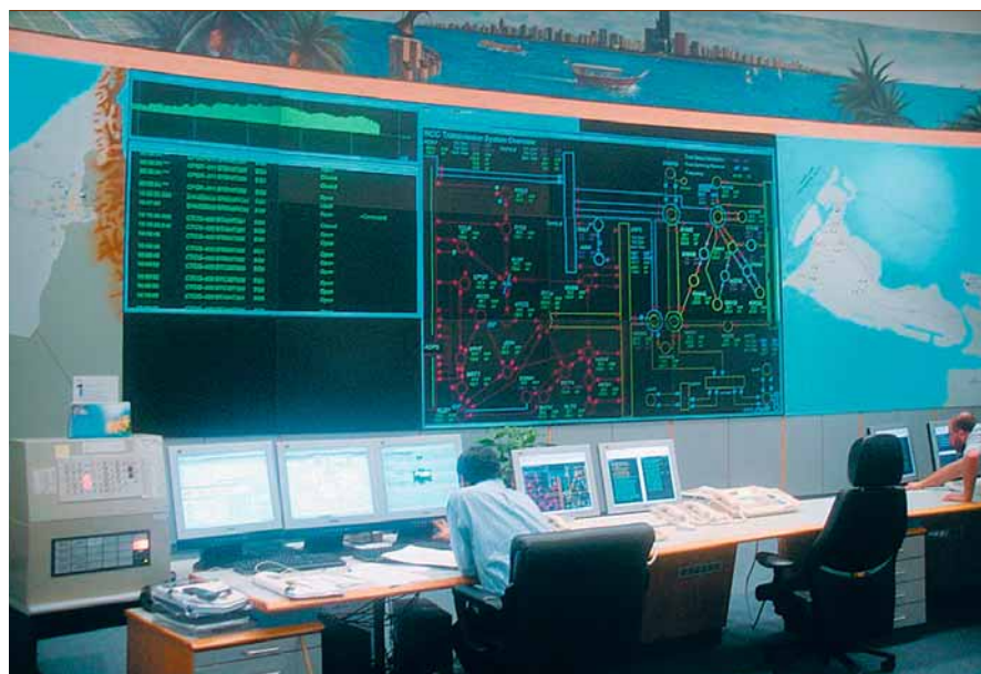
A typical control room
