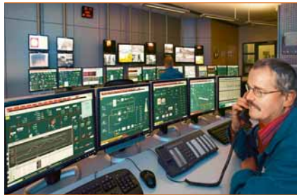
2 Control of a power plant to optimize production
