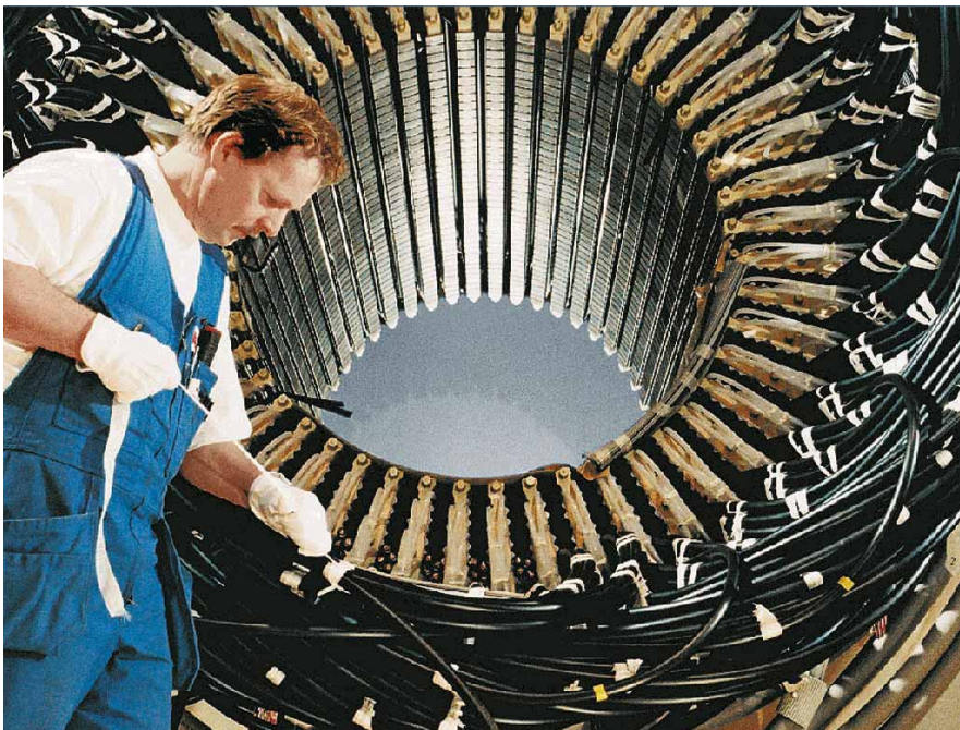
7 Cable-wound high-voltage motor as used to power the Troll platform in the North Sea
