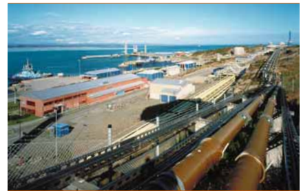
3 Obtaining the primary energy for electrical power generation
