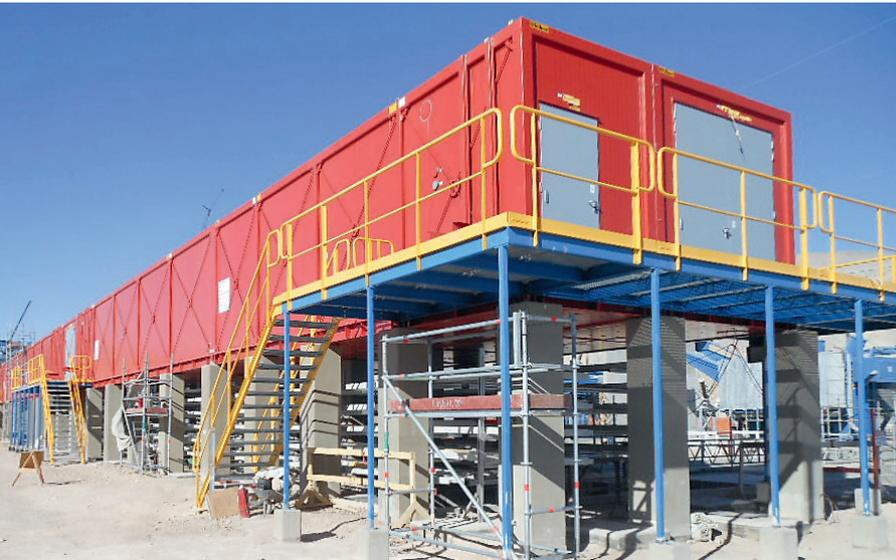
An E-house\* is a modular enclosure housing switchgear, variable speed drives, control systems and substation-related equipment. The flexibility of design means an E-house can be adopted for a wide variety of applications.
