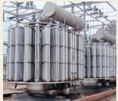
The three 9 MVA 22/66 kV GSU transformers are just as old as ABB Review . They were supplied by BBC in 1914.
