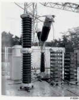
Fig. 1. Model assembly of an HVDC breaker developed by "Arbeitsgruppe HGU-Schaltan," in co-operation with Institut für Hochspannungstechnik der TU Braunschweig (the Institute for High-Voltage Technology at Brunswick, West Germany), undergoing tests at FGH, Mannheim-Phinzen, West Germany. From left to right: d.c. surge arrester, oil-immersion circuit-breaker and commutating capacitor.
