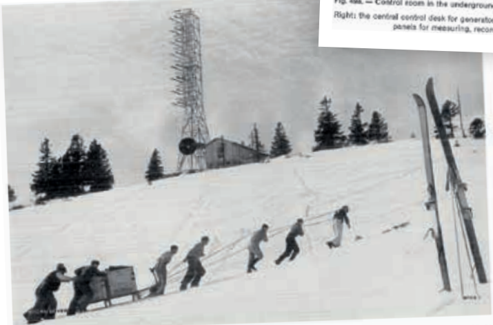
Fig. 5. — No machine could help on the last part of the way up to La Dôle television transmitter building which is at an elevation of 1800 m; muscular effort was the only way the separate sections of the vertical transmitter, weighing some 3 tons altogether, could be pushed up the mountainside.
