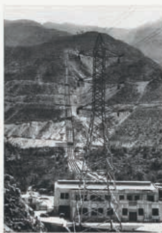
Fig. 1.— External view of the Juan Carosio hydro-electric power station, in Peru.
