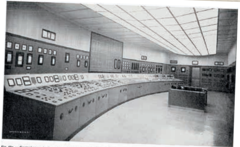
Fig. 496. — Control room in the underground power station of Santa Massenza, belonging to the Società Idroelettrica Sarca-Molveno, Italy. Right: the central control desk for generators, transformers and transmission lines; in the centre: the mimic diagram; and adjoining, the switch panels for measuring, recording, controlling and protection. Built by Tecnomasio Italiano Brown Boveri, Milan.
