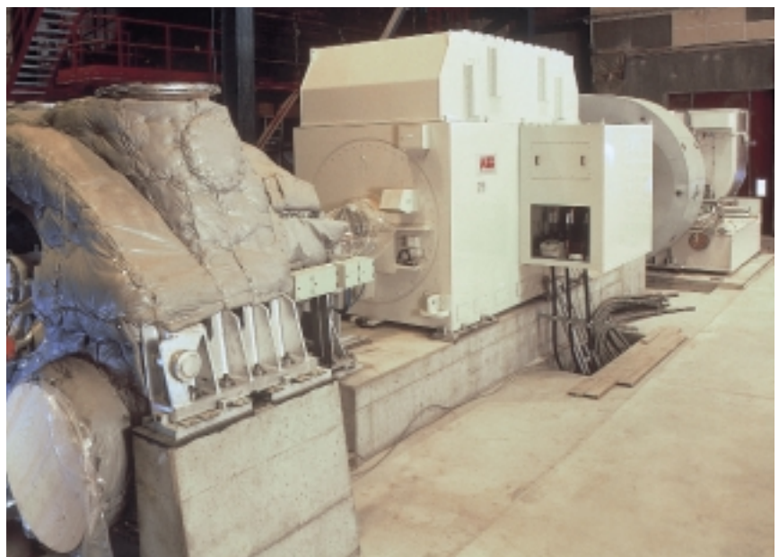
GT10 combined cycle, single-string installation 8
