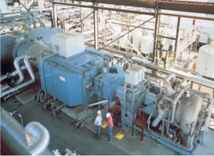
A VAX steam turbine installation with the high-pressure turbine and gear on one side of the generator and the low-pressure steam turbine and condenser on the other 11
