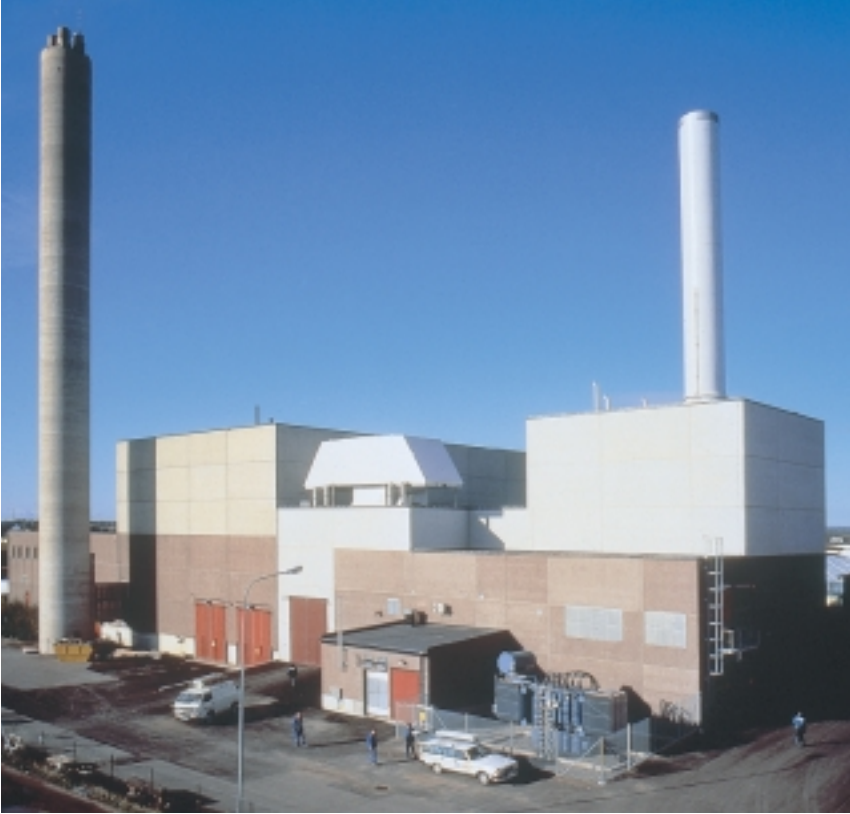
GT10 combined cycle plant at Ängelholm, Sweden
