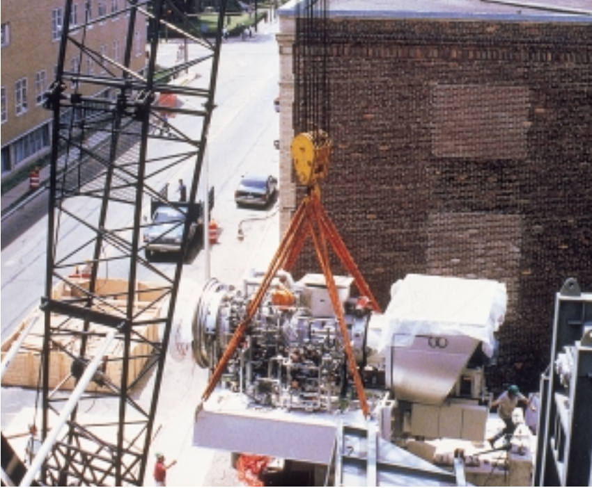
A GT10 gas turbine being lifted into an existing building on the premises of the Massachusetts Institute of Technology in Boston, USA. 7
