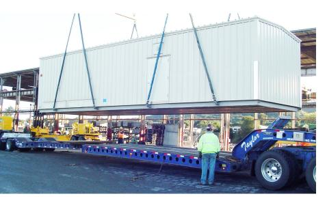
Electrification Services provides complete protection, automation, communication and control (PACC) systems for an entire substation, integrated into a modular building that is tested and delivered to site.
