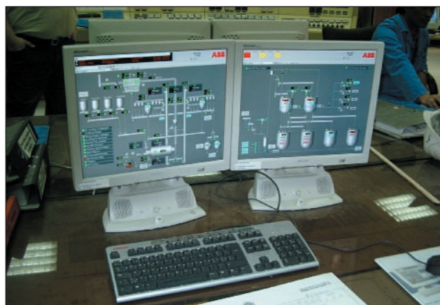
Operate IT process portal: a dualhead workplace.
