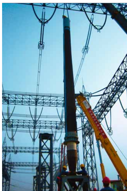
3 Installation of 1,100 kV AC bushing (2008)
