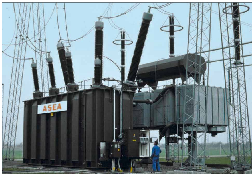
800 kV DC converter transformer (2008)
