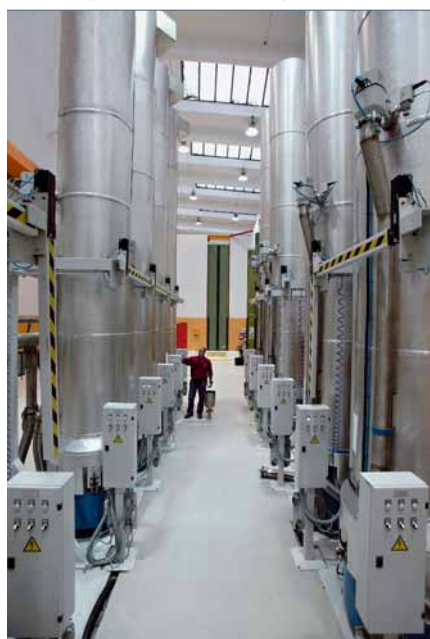
2 Impregnation of RIP bushings
