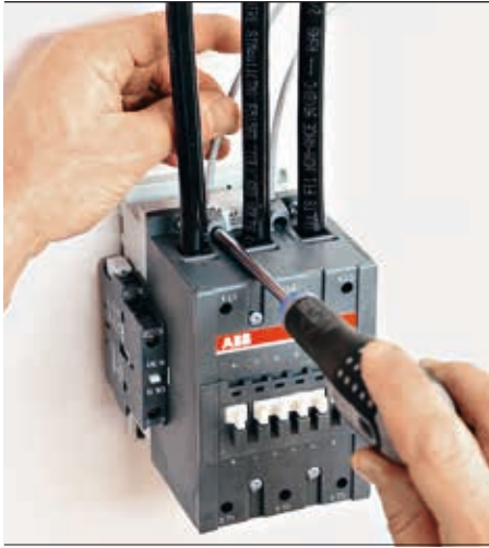
2a Older contactor with main circuit in the front
