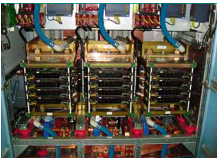
7 Inverter unit of ACS6000 frequency converter
