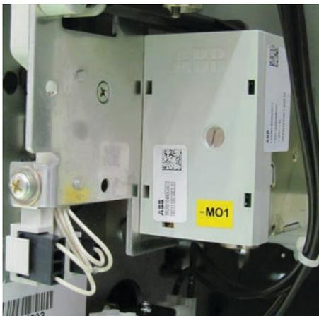
Allows the device to be opened by remote control.
