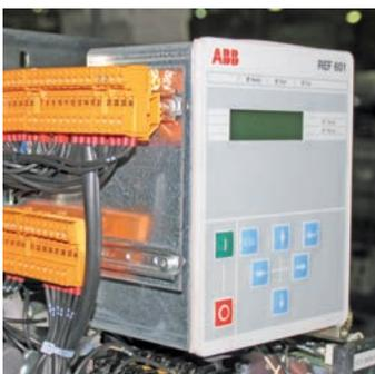
REF 601 relay coordinated with circuit-breaker and with the current sensors
