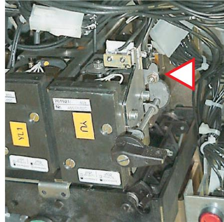
Overrides the mechanical action of the undervoltage release (4), allowing the circuit-breaker to close with the undervoltage release de-energized. It is always fitted with electrical signalling of release excluded.
