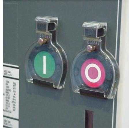
Allow the circuit-breaker's operating mechanism knobs to be locked.
