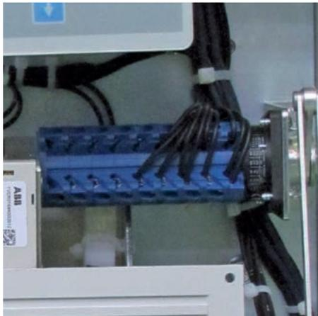
The standard equipment includes a set of five auxiliary contacts. Other additional sets of auxiliary contacts are available on request, with a surcharge. Their number depends on the version of the device. See summary of the total quantities that can be supplied.
