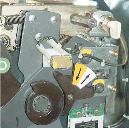
Installed in an electric circuit, this signals the state of the operating mechanism's closing springs.
