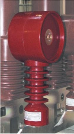
The current sensors transmit the current signal to the relay for processing and provide the energy to power the relay and opening solenoid if tripping occurs.
