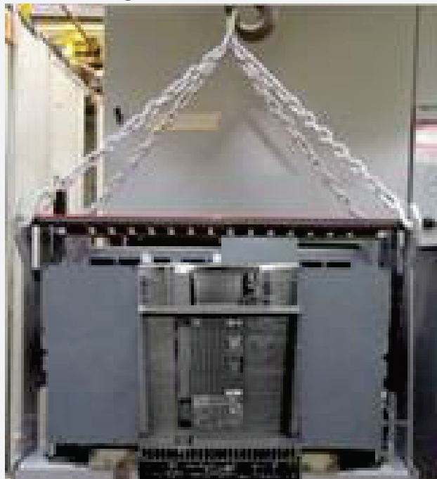
AKD-8 Using Chain & Hook (alternate method)
