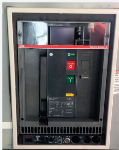
Emax 2 Retrofill , AKD-8, Connect Position
