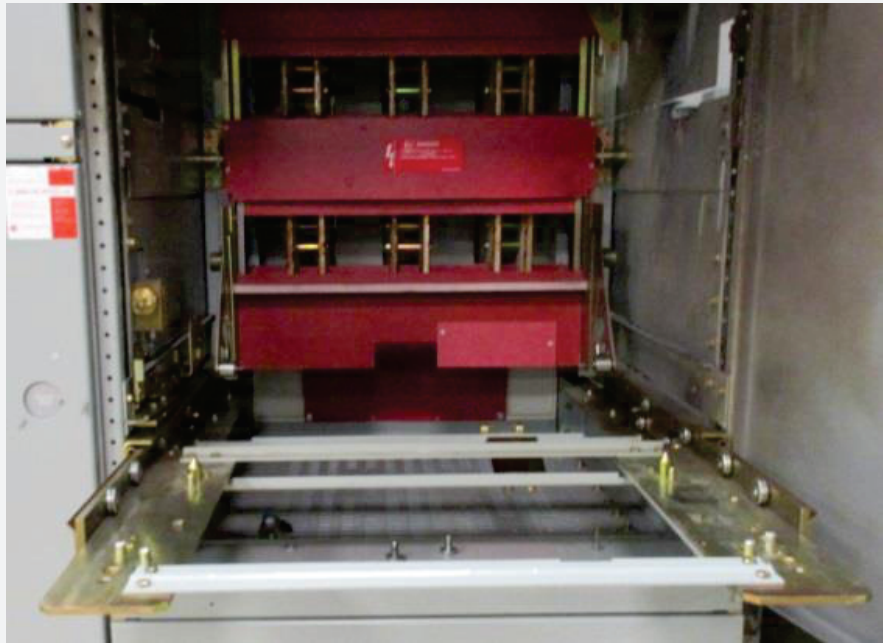
AKD-8: Empty Compartment, View 2, Drawout Tray Extended
