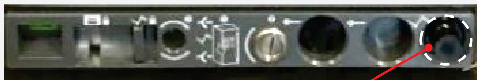
AKD-8, Racking Tool & storage location
