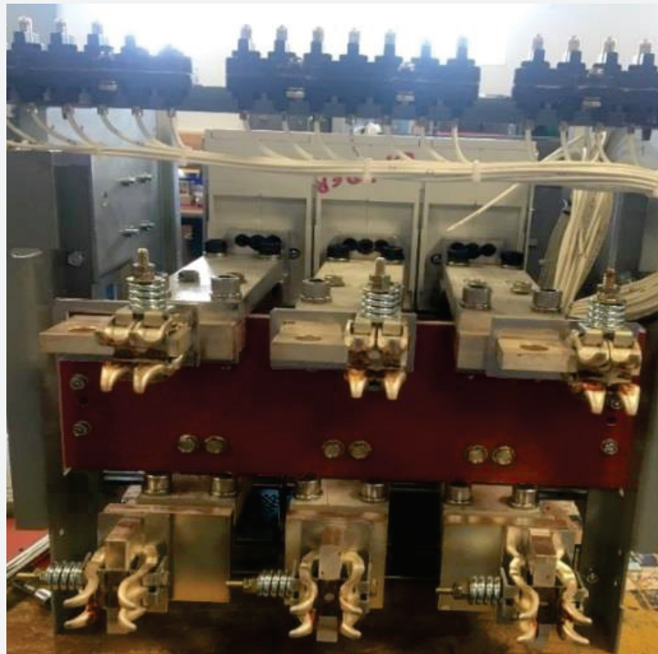
AKD-8 Primary Contacts or “Fingers” (Apply Grease to sliding surfaces)
