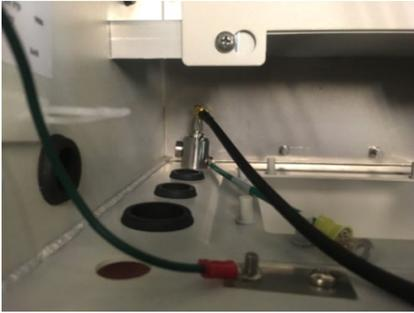
17. Attach the ground cable to the ground post (see number 2 in the picture below).
