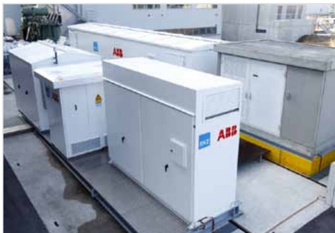
The complete package: PCS100 ESS converter, LG battery, switchgear and transformer
