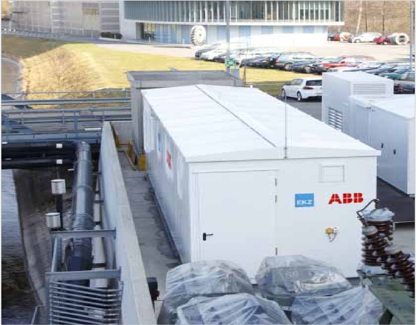
PCS100 ESS 1 MW / 500 kWh battery solution at the Dietikon Powerplant based in Switzerland
