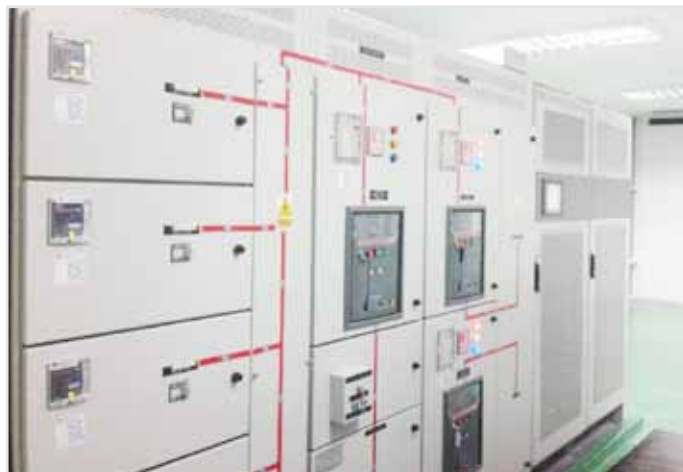
PCS100 AVC installation in a temperature controlled room
