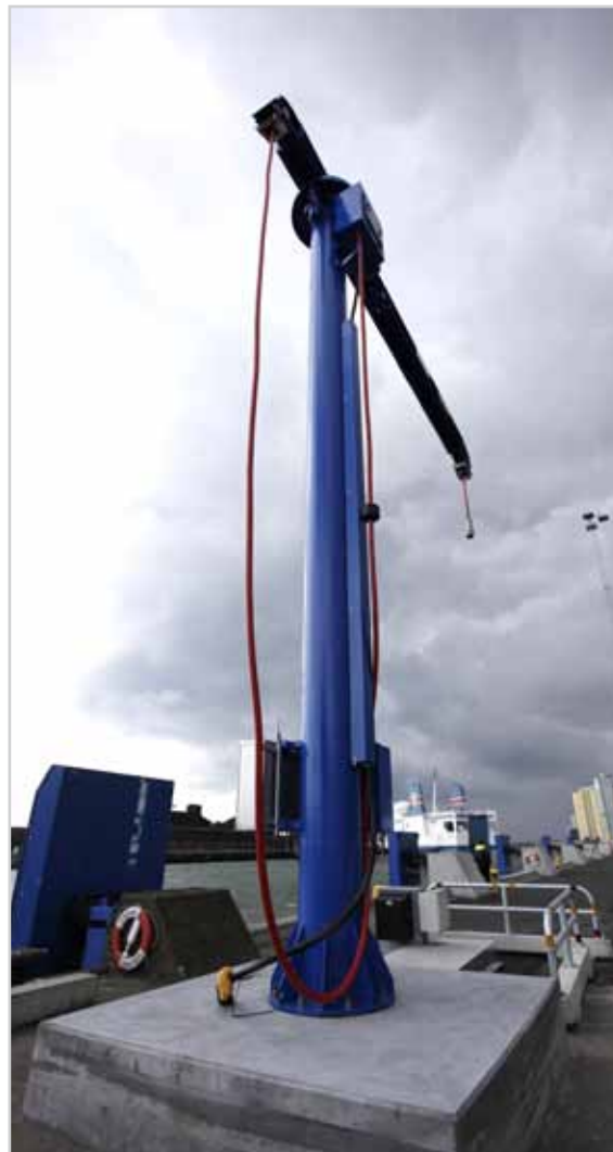
One of the cranes enabling the shore-to-ship connection
