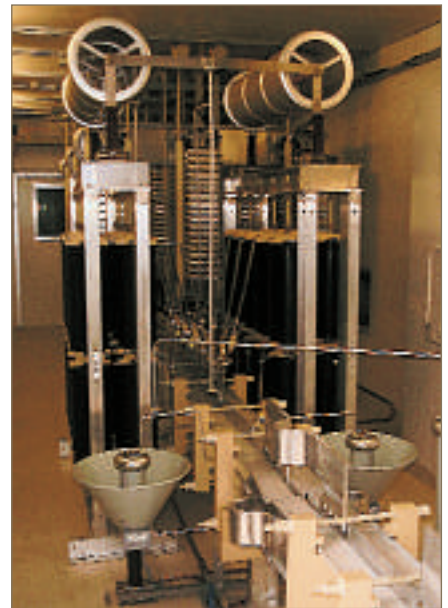
DC-link capacitor bank with the new dry HV capacitors, here in an HVDC Light converter module
