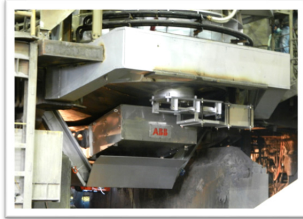
Figure 1. Arc Furnace with stirrer mounted underneath the furnace bottom at SDI site.
