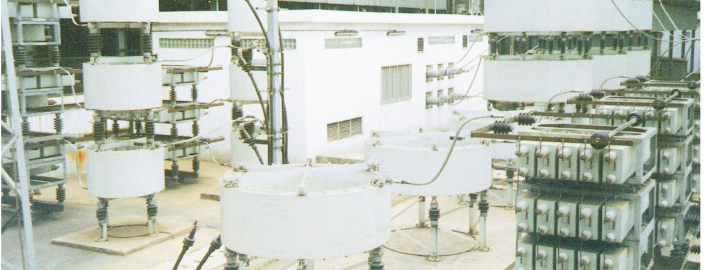
A Static Var Compensator (SVC) rated at 2 Mvar inductive to 56 Mvar capacitive at a voltage of 22 kV supplied by ABB is in operation since 1993 in the NatSteel steelplant in Singapore. The purpose of the compensator is to provide dynamic control of reactive power, power factor correction and reduction of fast voltage variations created by the simultaneous operation of electric arc furnaces of DC and AC type in several possible combinations:
