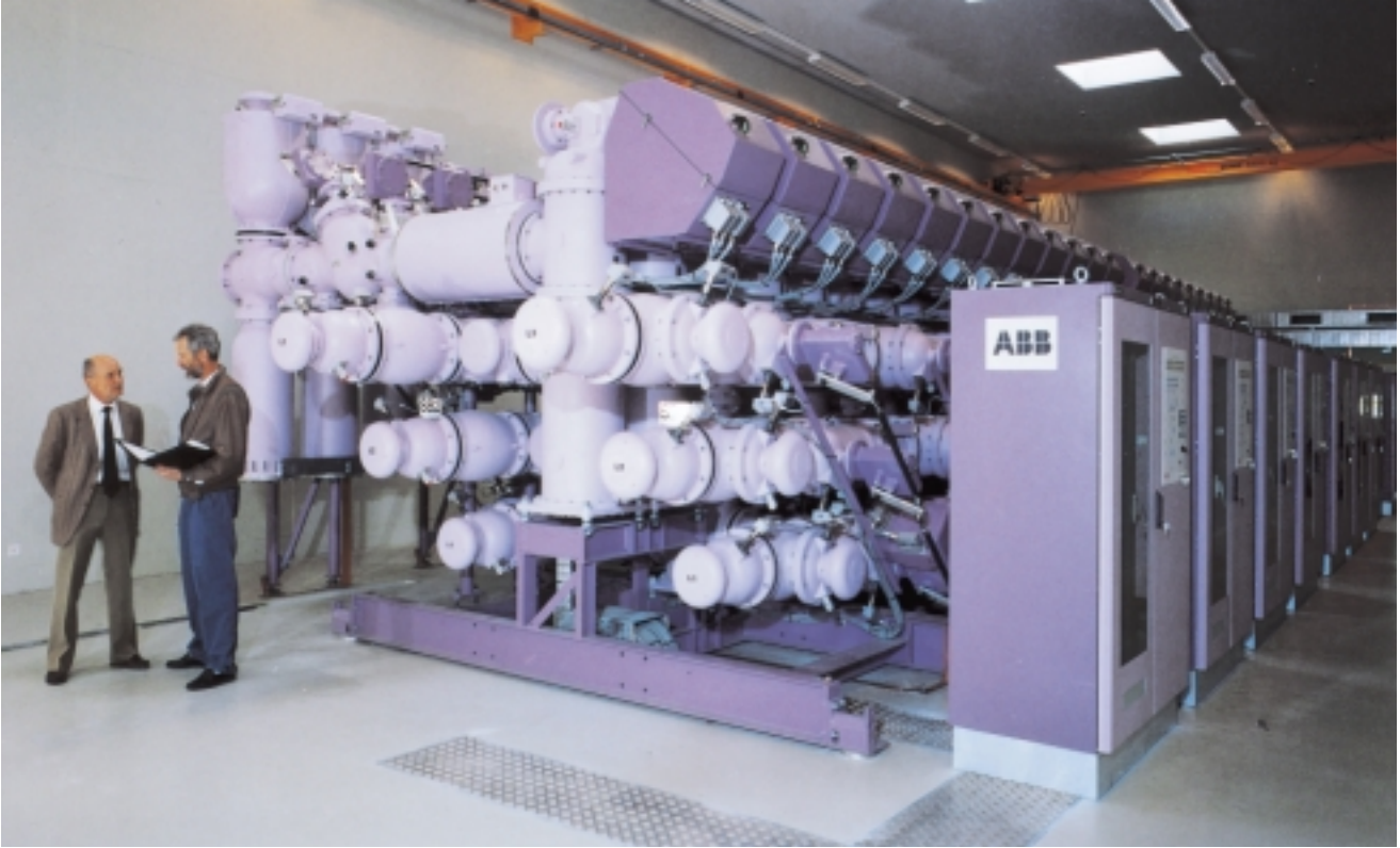
Example of a modern 300-kV gas-insulated substation with integrated cubicle for the control and protection equipment 1
