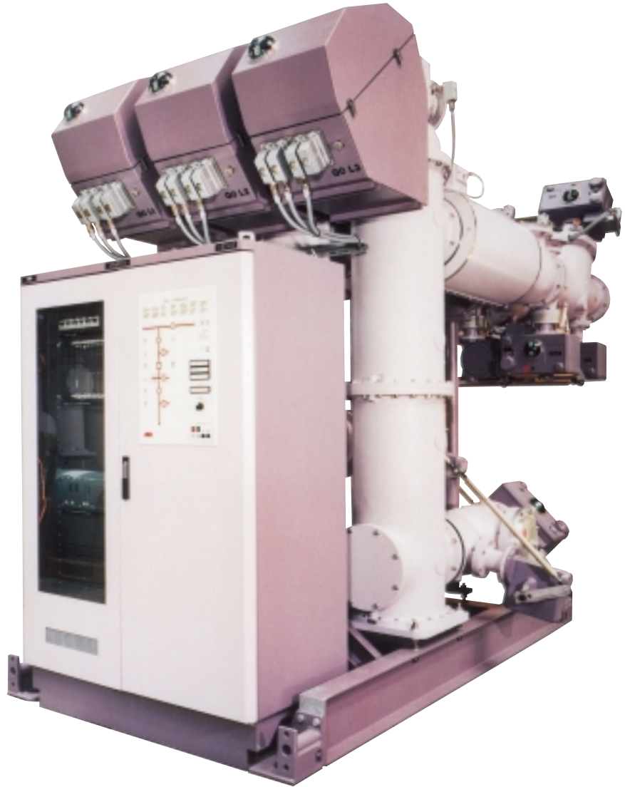
GIS bay with modern integrated control cubicle
