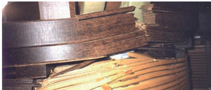
Failure mode: collapse of end support.
