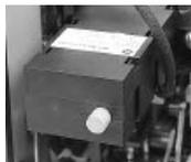
The bell alarm device is provided with two C-form contacts – each C-form contact is 1NO and 1NC contact with a common connection. The bell alarm device operates whenever the breaker trips due to a protective function of the trip unit. It can be used to provide remote indication of a fault trip and/or disable electrical operation of breakers that may have automatic control.
