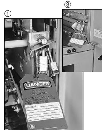
This array of locking features should accommodate any type of “lockout - tagout” procedure a customer may have implemented at their facility. All of the padlock provisions on WavePro breakers and AKD-10 equipment will accept any combination of up to three padlocks with 1/4" to 3/8" diameter shank.
