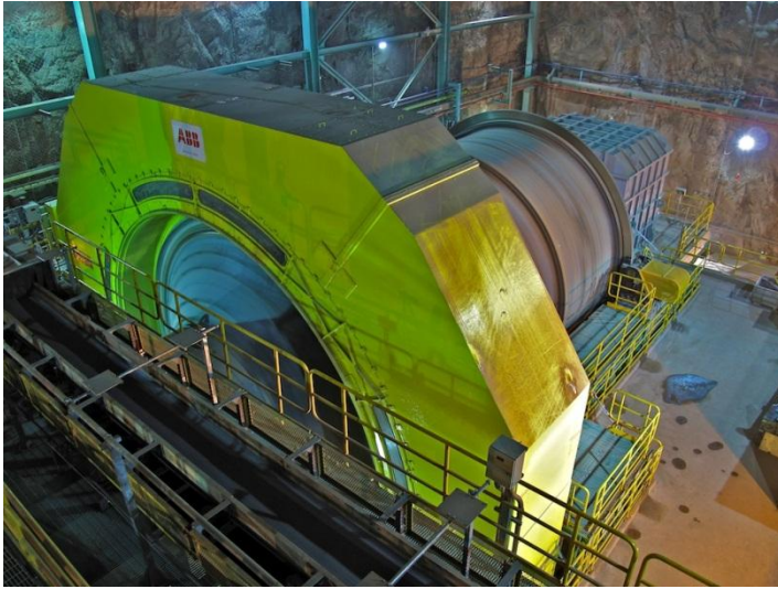
Gearless mill drive
