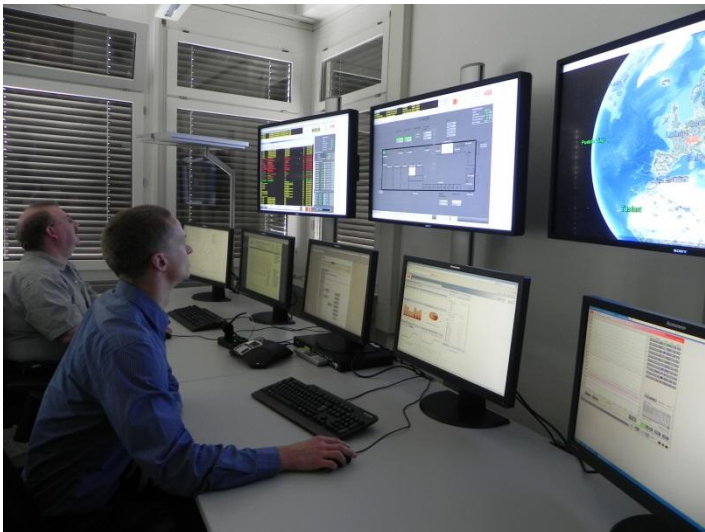
ABB remote control room
