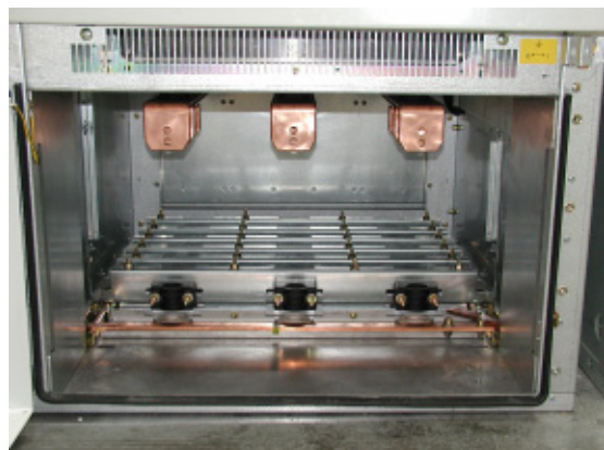
6 cables per phase 1000 mm wide unit
