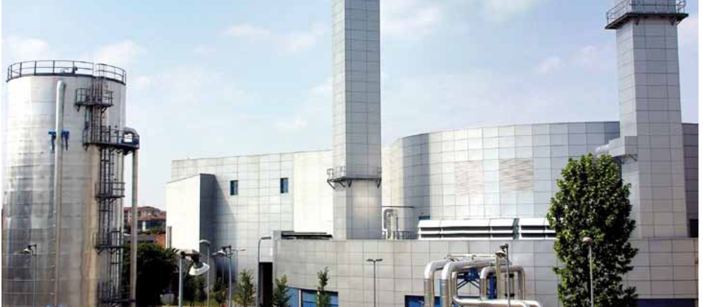
Canavese district heating plant, Italy
