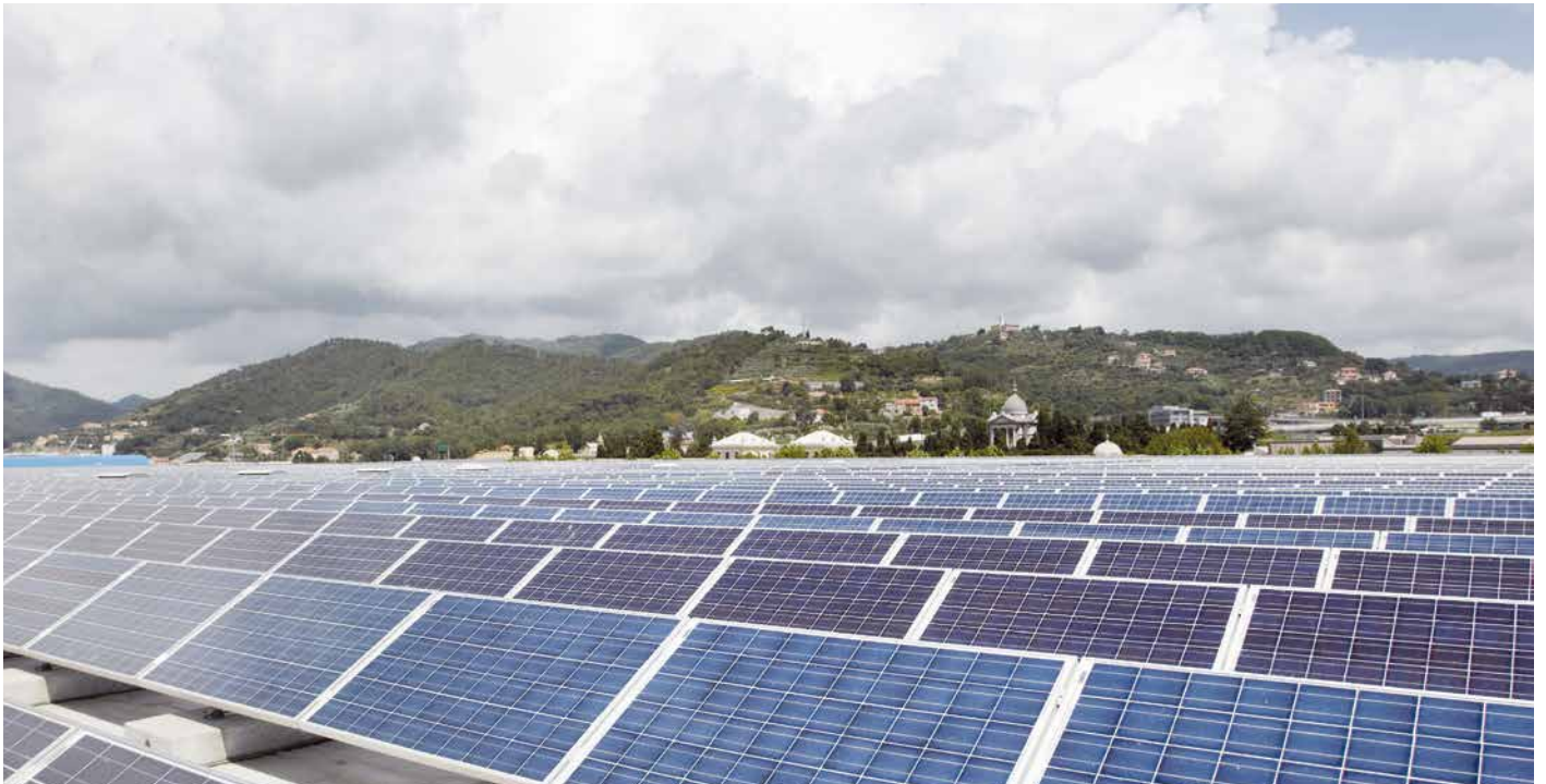
GFDI - Ground Fault Detection Interruption (48)
