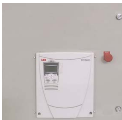
TYRAK L control cubicle door with mounted DCS800-R
