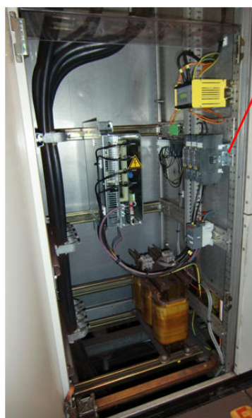
Field exciter with auxiliaries in AC-Incoming
