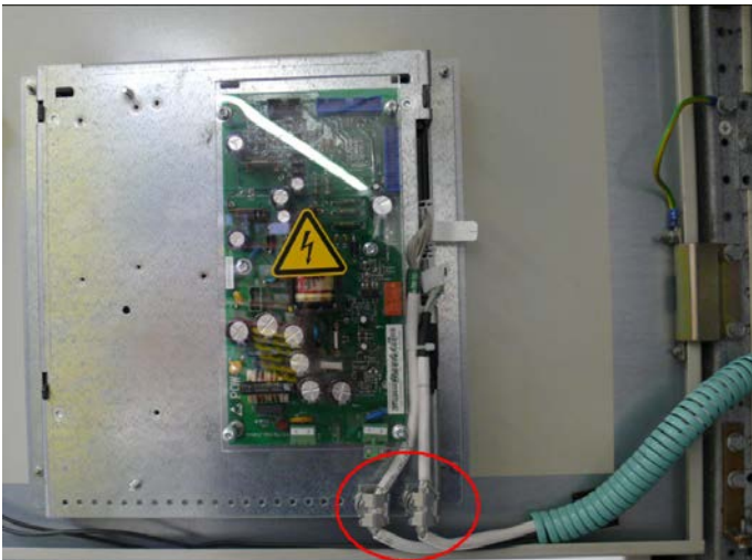
Screening the flat cables
