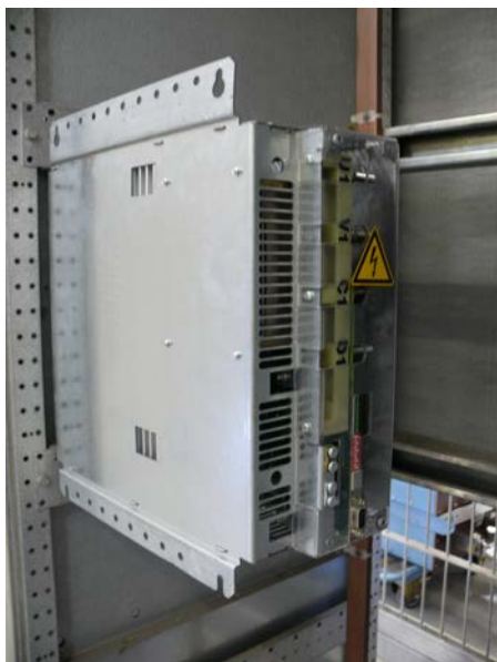
DCF503-0050B mounted to existing DIN rail in AC-Incoming
