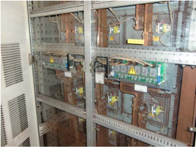
Installed PIN-48 Mounting Kit4Q (Power stack)
