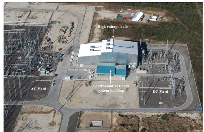
Figure 1. Aerial view of HVDC converter station.
