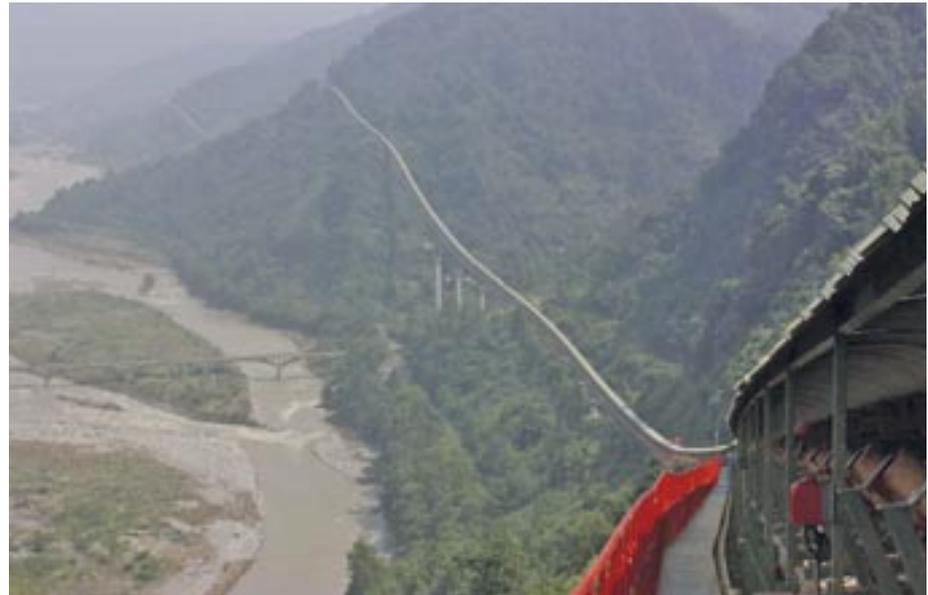
structure of the premises. They are also able to safely handle steep sloping routes, rivers or road crossings. The system provider determines the optimum conveying route, then takes over project planning and installation. BEUMER Group also ensures that the owner remains sustainably competitive - with cost efficiency and comprehensive customer support.
