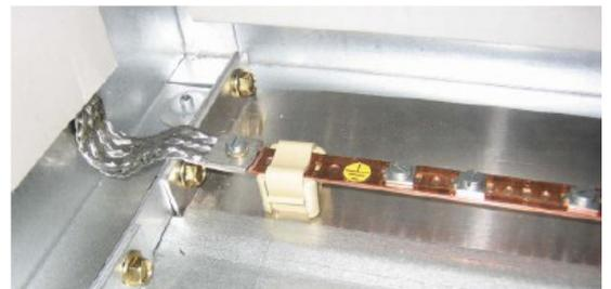
Figure 73: connection to the busbar in an MV panel
