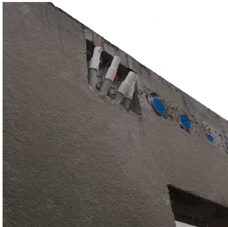
Conduit end piece in the front surface of the prepared element.
