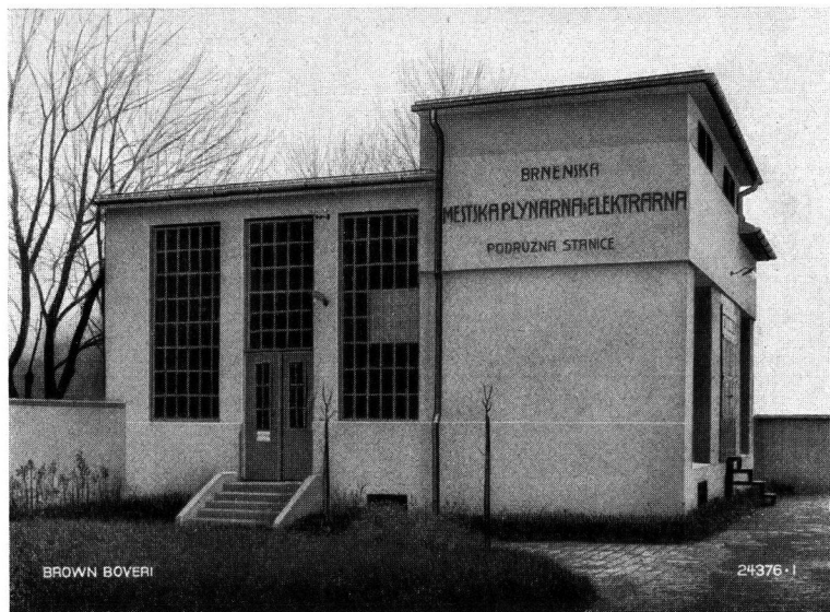
Fig. 9. — Exterior view of Sebrowitz Substation of the Brno Tramways.
