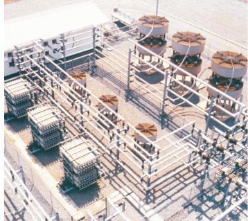
The SVC control system is built up by micro-processor based computer functions that constantly monitor the status of the SVC reactive output and status of switching devices. It comprises a voltage regulator based on closed-loop three-phase symmetrical voltage control.
