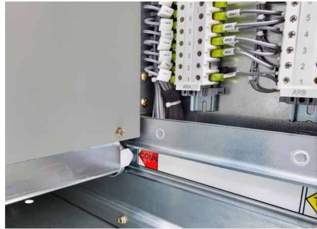
Figure 4.24 Circuit breaker in CONNECTED position
