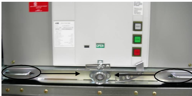
Figure 4.10 Truck handle actuation
