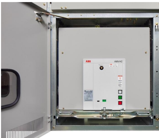
Figure 4.21 Circuit breaker in DISCONNECT position
