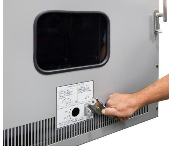
Figure 4.22 Racking release handle
