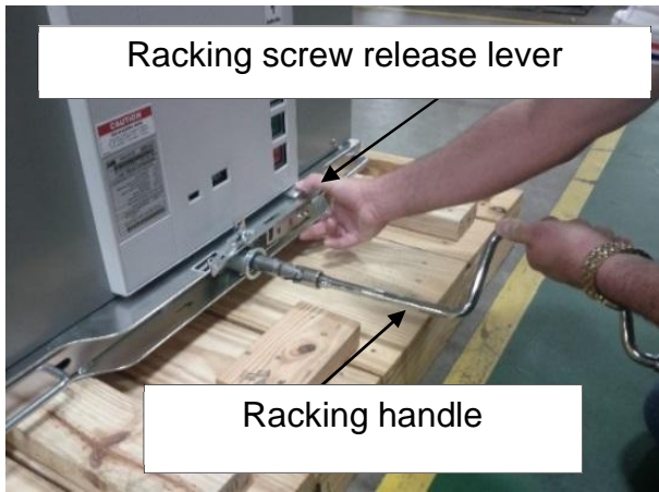
Figure 4.8 Truck racking screw
