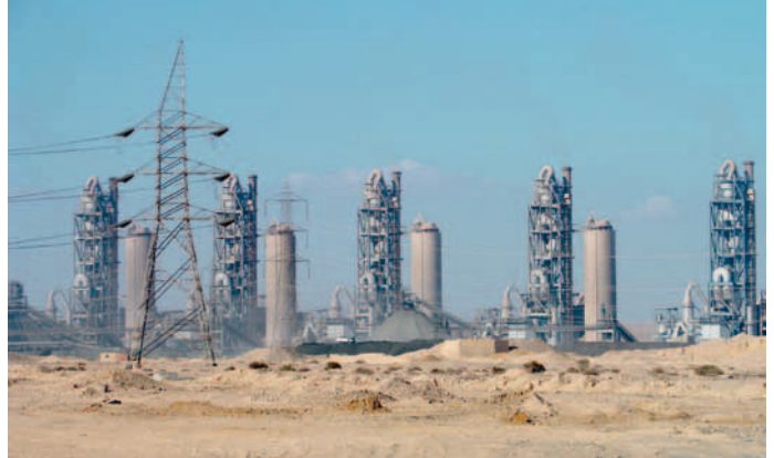
ECC Lafarge plant in Ain Sokhna
