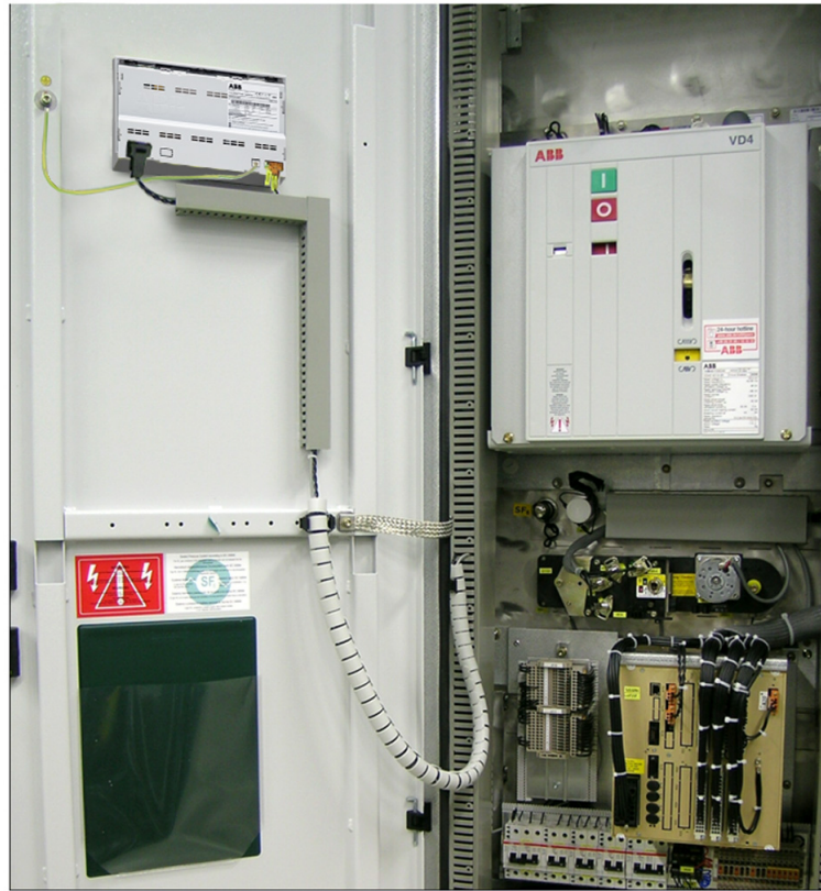
Fig. 3.-3 Mounting of the central unit in the LV compartment and the HMI on the door
