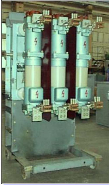
Retrofit of Russian switchgear by replacing the air breaker with vacuum circuit breaker type VM1
