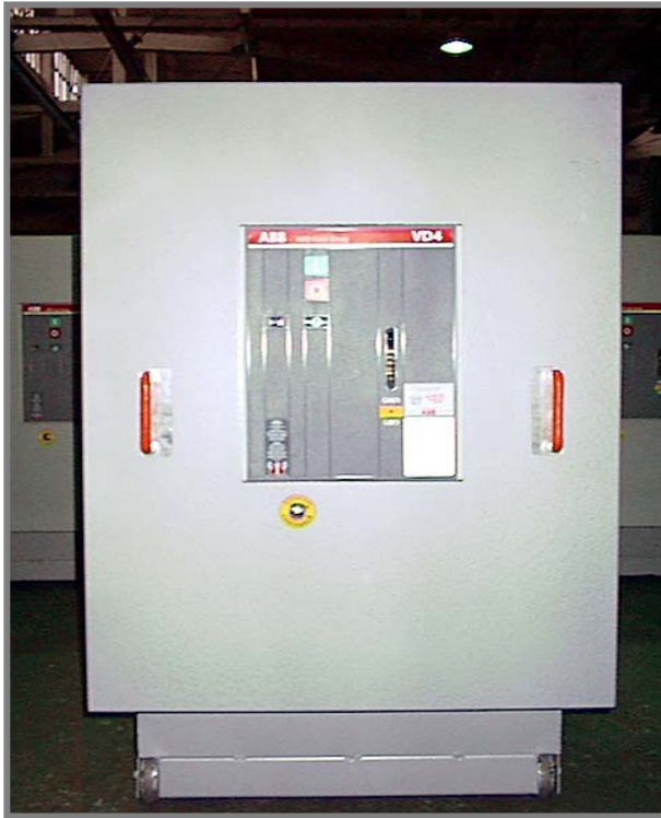
Retrofit of polish switchgear by replacing the oil - minimum breaker with vacuum breaker type VD4
