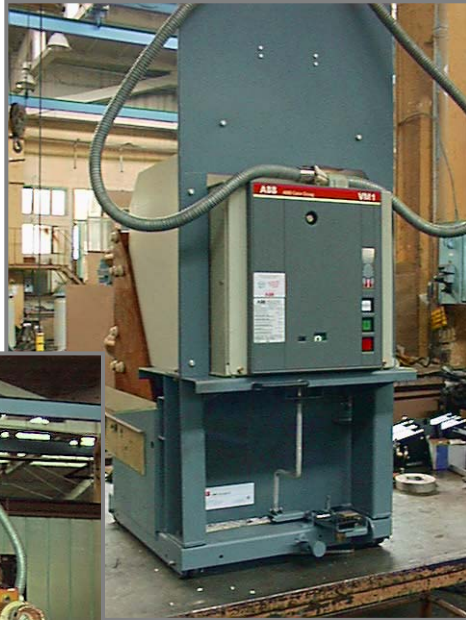
Retrofit of Russian switchgear by replacing of the airblast breaker with vacuum breaker type VM1
