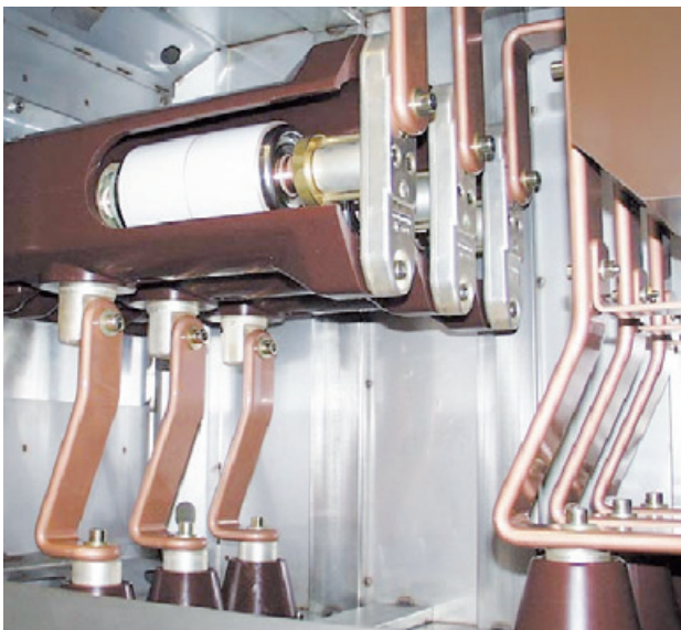
Fig. 7.1.1: Vacuum circuit-breaker
