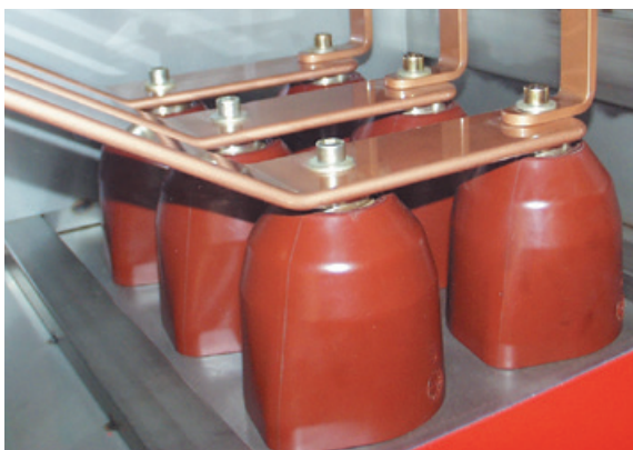
Fig. 7.4.1: View into the gas-insulated circuit-breaker compartment with inner cone sockets
