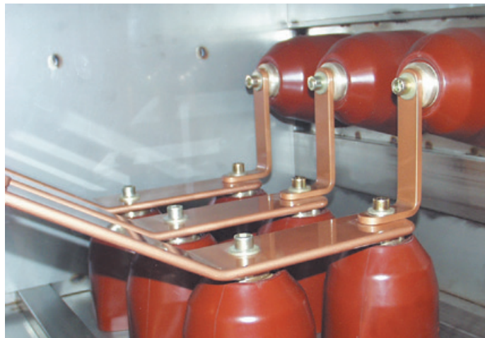
Fig. 7.6.1: View into the circuit-breaker compartment: test sockets
