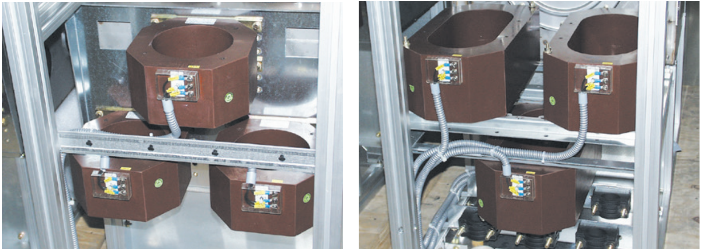
Fig. 7.8.2.1: Ring core current transformer
