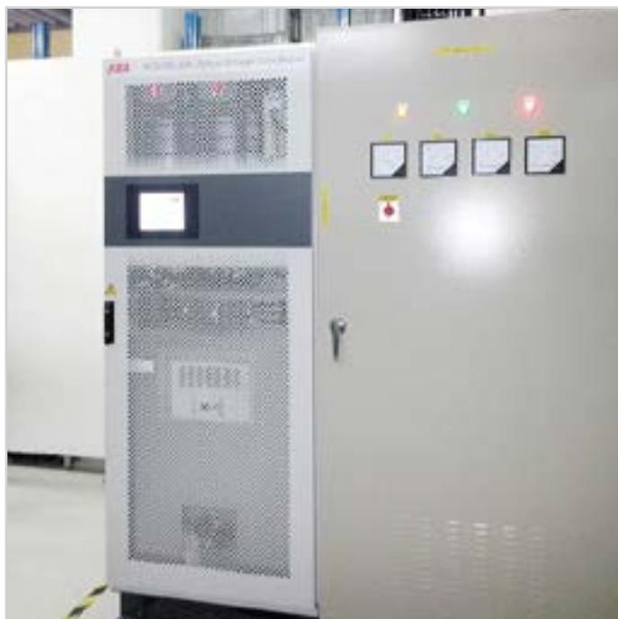
ABB's 300 kVA PCS100 AVC to ensure HHGrace is protected against power disruptions
