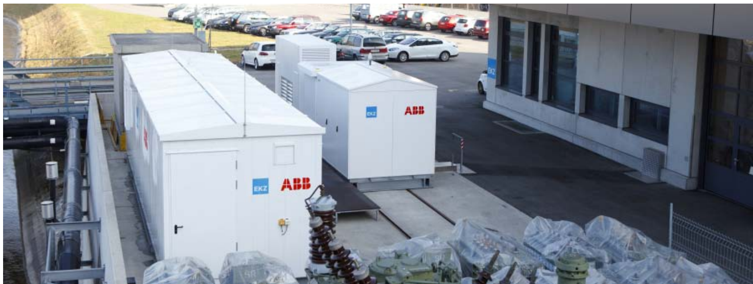
BESS 1 MW / 250 kWh PCS solution at the Dietikon Power Plant in Zurich, Switzerland.
