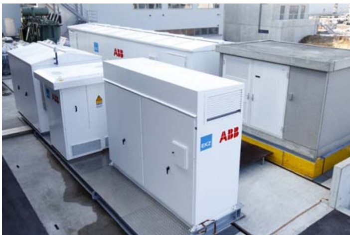
The complete package: PCS package, LG battery, switchgear and transformer
