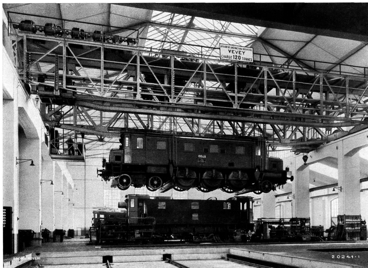
120-TON LOCOMOTIVE CRANE AT THE YVERDON REPAIR SHOPS OF THE SWISS FEDERAL RAILWAYS.
