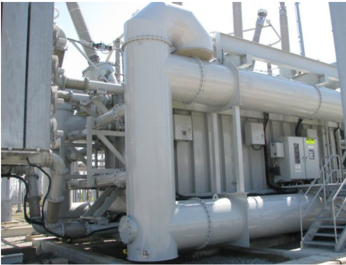
Figure 1: Transformer with pressure relief system (left) and flexible tank design (right)
